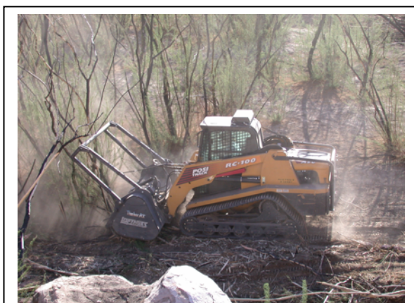
Clearing tamarisk with a Timber Axe mastication head
